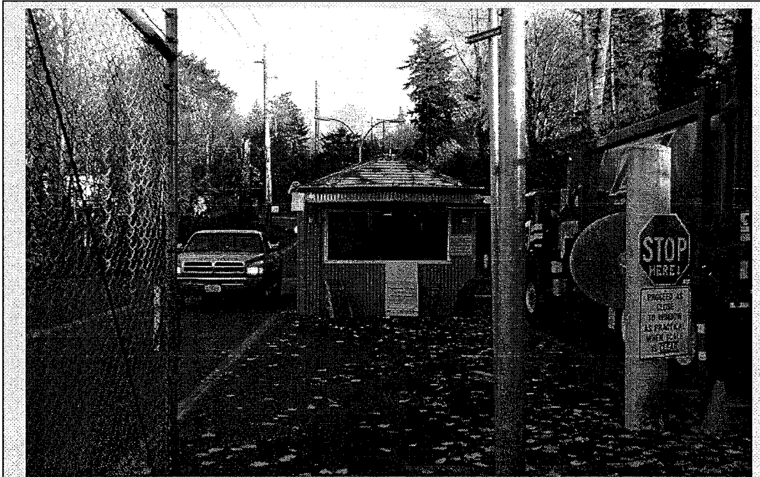
Photo 1. View of scalehouse at entrance
